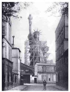
The 151-foot-high statue was prefabricated in Paris by molding sheets of copper over a stainless-steel framework. The picture (*left*) shows Liberty towering over the buildings in Paris. The builders had to be sure all the pieces fit so they completely assembled the statue, then took it down and shipped the pieces to the United States in 214 crates in 1885.
