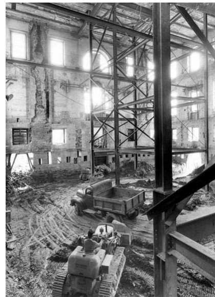
White House reconstruction, 1948-1952
